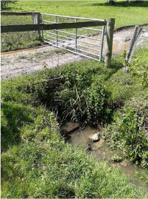
Graphic 4-17 Culvert Chancton Farm stream
