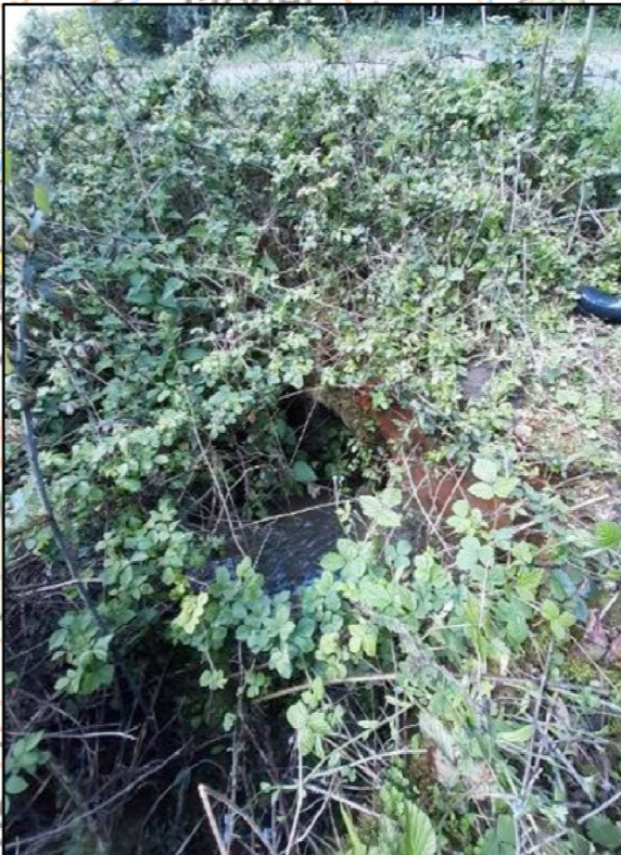
Road culvert, Washington road
