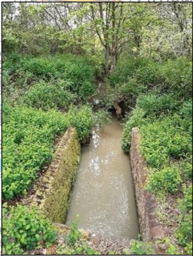
Onshore cable crossing site STRX-15
