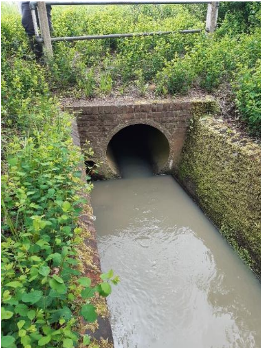
Graphic 4-45 Road culvert upstream of proposed cable crossing site STRX-15
