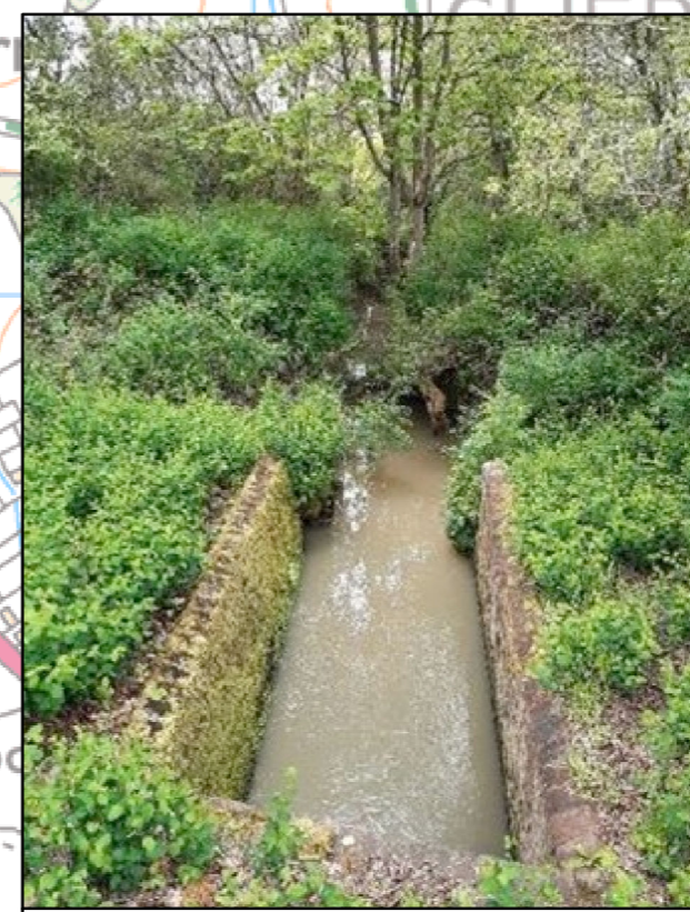
Cable crossing at site STRX-16
