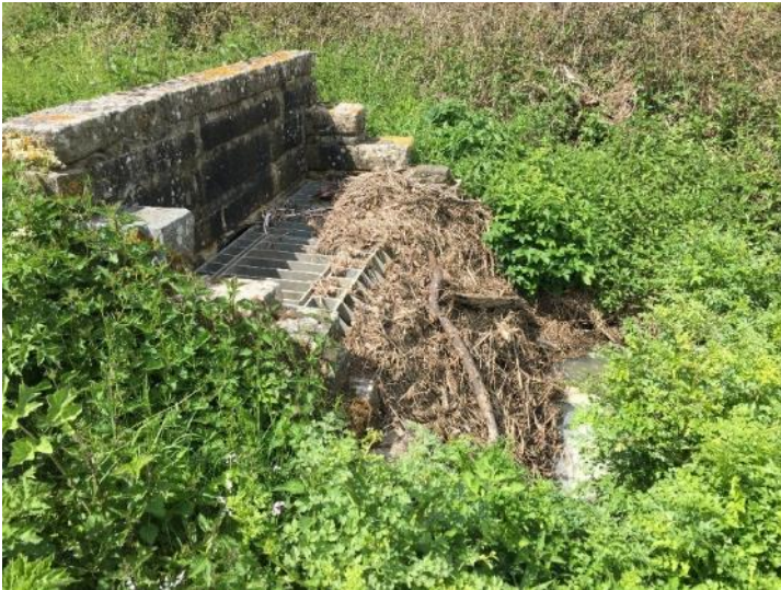
Graphic 4-12 Heavily fouled coarse screening on the downstream entrance to the A283 road culvert at Washington, West Sussex immediately upstream of the proposed crossing site STRX-02
