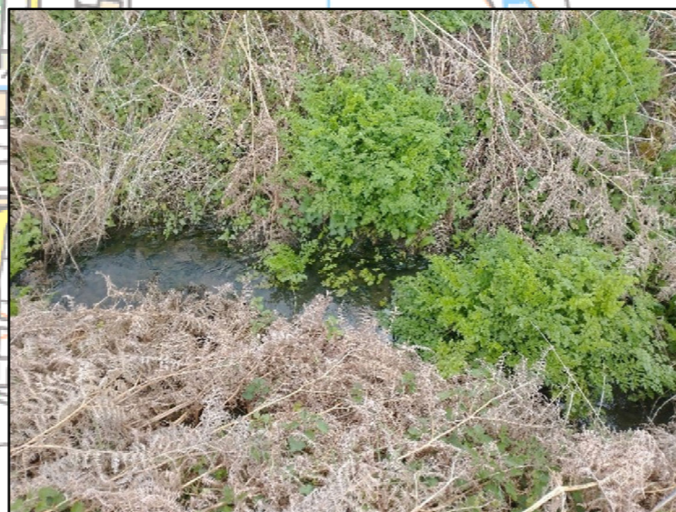
Onshore cable crossing DTX-14
