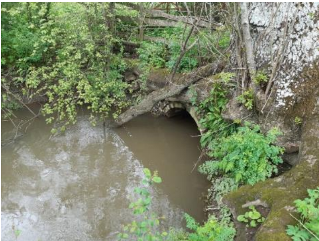
Graphic 4-48 Farm crossing culvert upstream of site STRX-18
