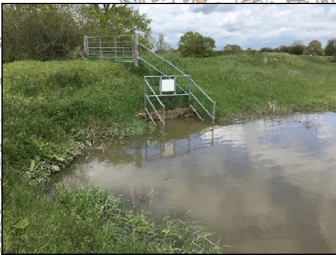
Culvert and tidal flap at confluence with River Adur
