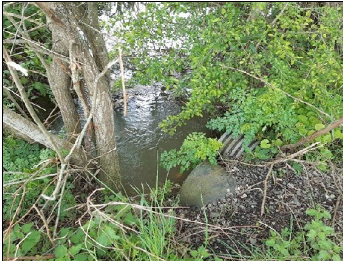
Twin pipes at inlet to downstream lake
