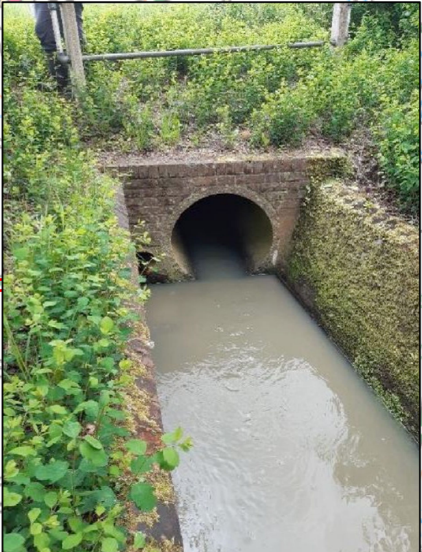
Road culvert upstream of proposed cable crossing site STRX-15
