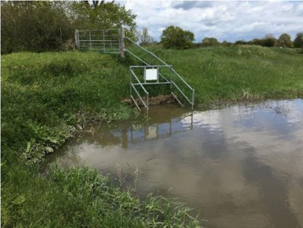
Graphic 4-41 Culvert and tidal flap at confluence with River Adur
